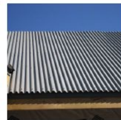
9 MRVMCR, GALVANISED CORRUGATED ROOF Paint finish. Clear anti-graffiti coating.
