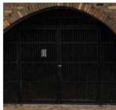
2 XMG, EXISTING METAL SCREEN AND GATE
