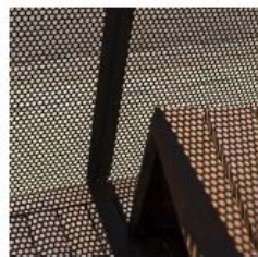
7 MOP, PERFORATED METAL SCREEN Approx. 50% open area. Paint finish. Colour similar to Colorbond Monument.
