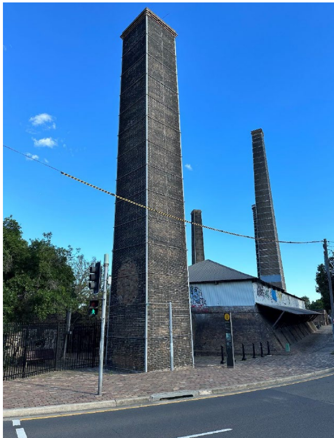
intersection of Princes Highway, Sydney Park Road and King Street
